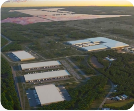
Data Center Project at Astra Enterprise Park in De Soto, Kansas
