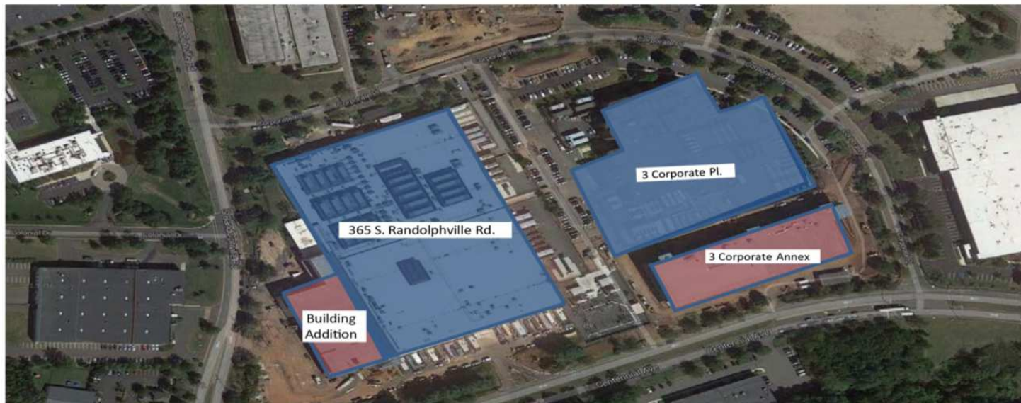
Completed and Stabilized Development Current Development
