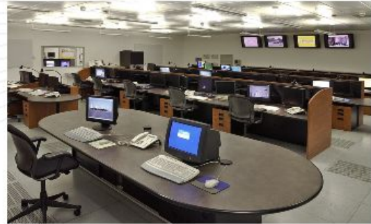
Systems and security controls
