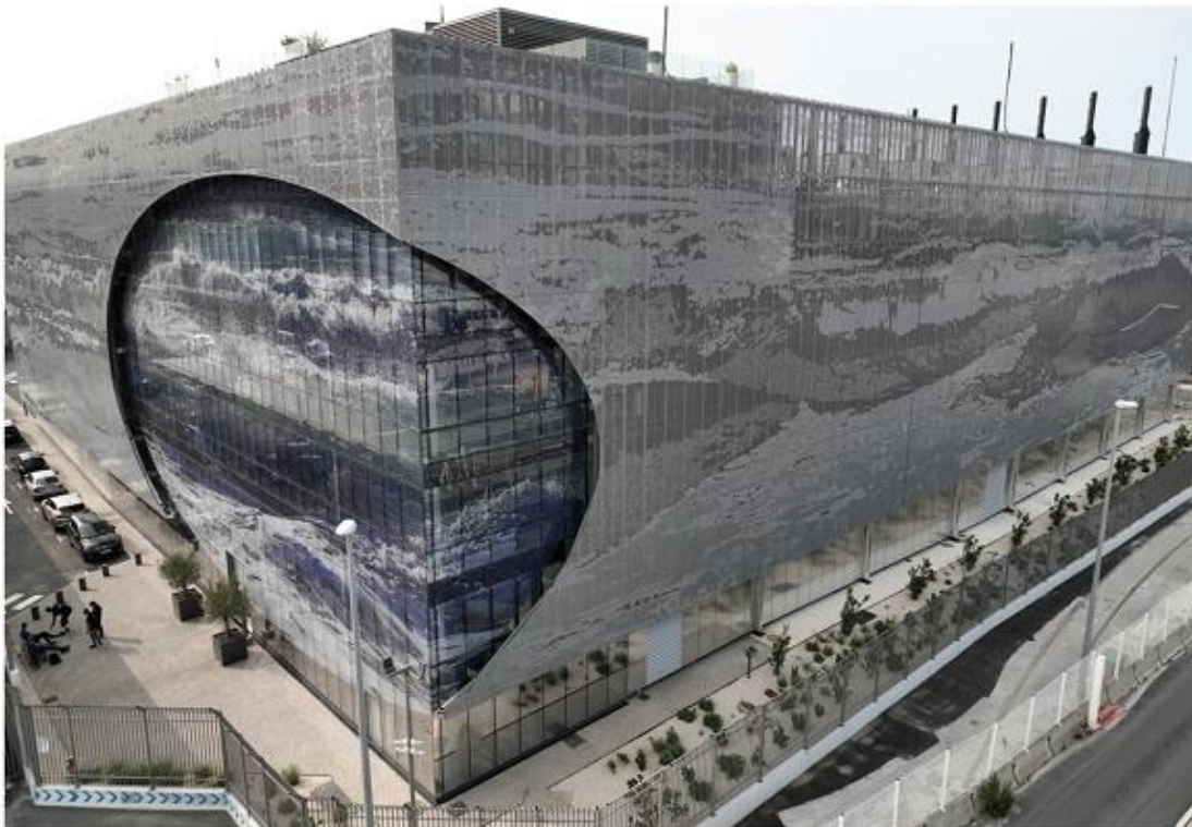
Located in Marseille, France, MRS4 is built on the site of former industrial warehouses, which are part of the Grand Port Maritime de Marseille.
